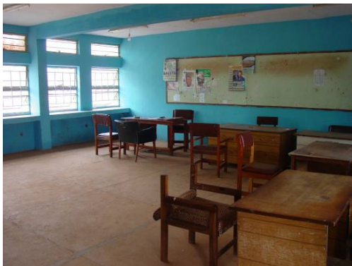
A typical room used for administration. Note the broken furniture, but also the unused space – raising a challenge as to whether existing facilities could be used more efficiently and whether repairs could be done locally.
